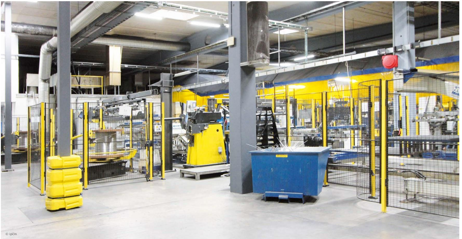
The machine guarding solutions from Axelent protecting its own manufacturing department.
