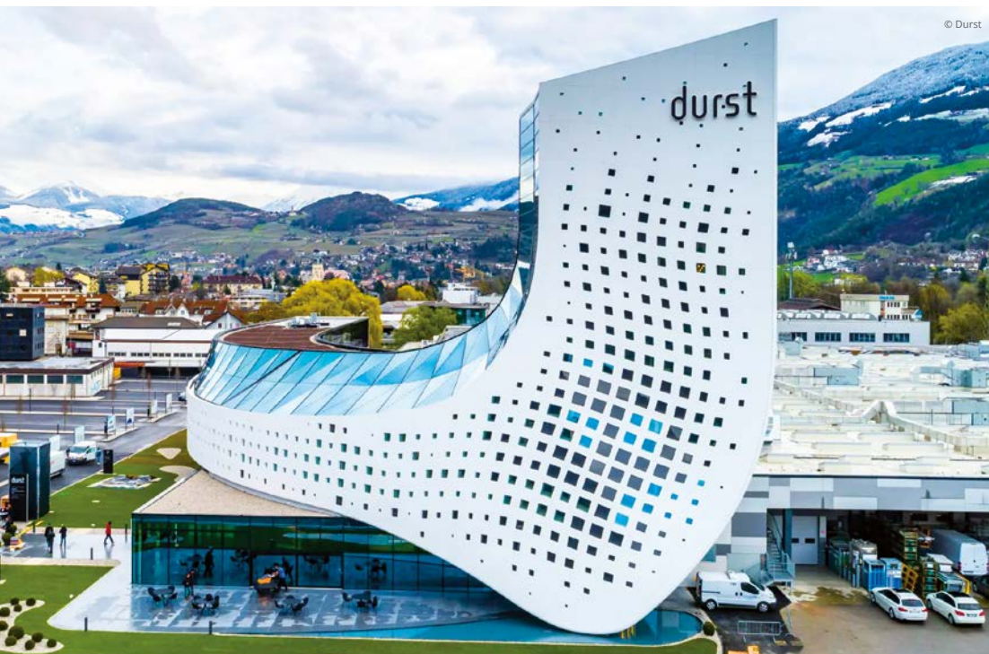
Durst's headquarters in Brixen: in 2019, Pintarelli Verniciature powder-coated the aluminium components of its façade in compliance with the QUALICOAT certification standards.
